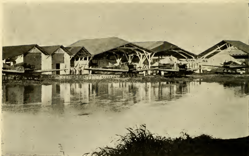
THE HANGARS IN BARRANQUILLA
